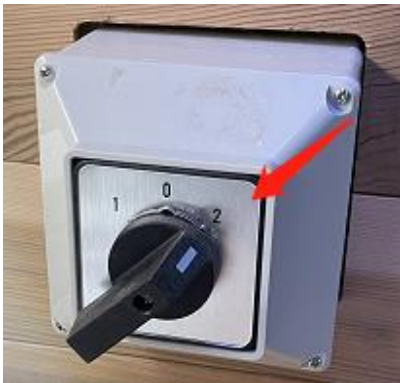
Power to Infrared heaters
