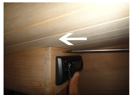
FIG-15.4 Screw wood housing to sauna room
