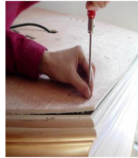
FIG-18.1 Screw down Roof Cover
