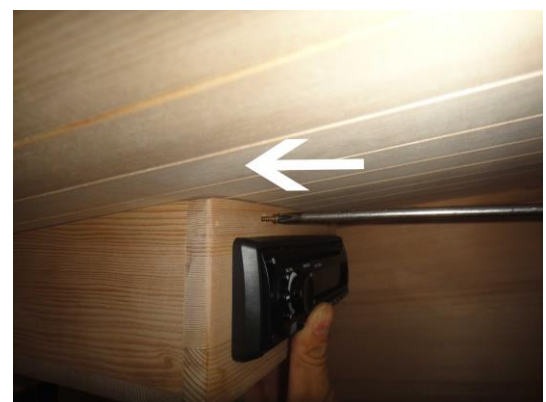
FIG-15.4 Screw wood housing to sauna room
