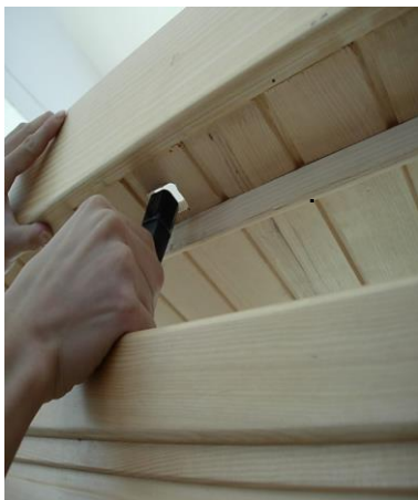
FIG-12 Slip cords/wires through corresponding holes
