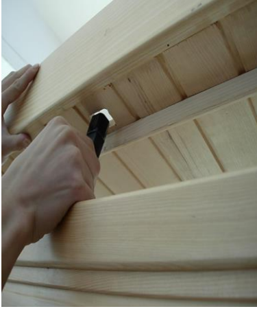
FIG 12 Slip cords/wires through corresponding holes
