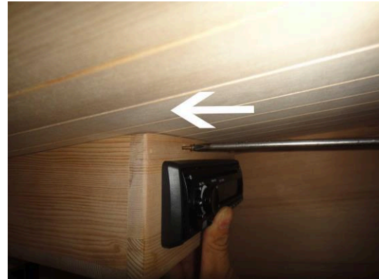
FIG 15.4 Screw wood housing to sauna room
