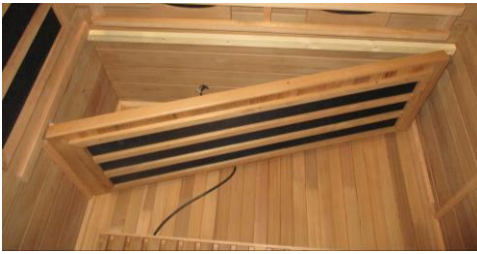
FIG-9 Installing Bench Heater
