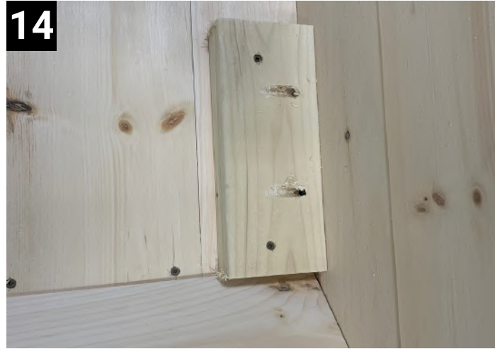
14 Screw down floor cleats then push down on wall board so it's tight to floor then put in the 2 pocket screws.
