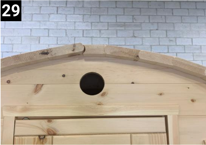
29 Set top stave in and then close up staves tight. Screw all staves down with screws now
