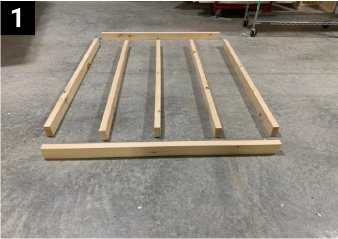
1 Floor base. On level surface screw 5 long boards with the 2 56" end boards
