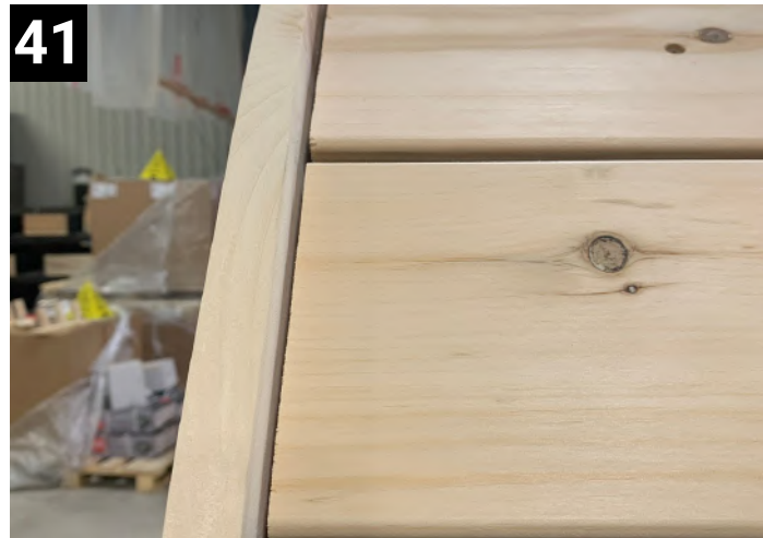
41 Keep ends even with barge boards to look nice
