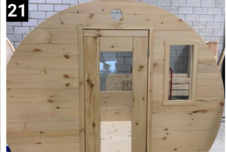
Put top pc of wall over door and fasten with 4" screws
