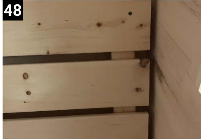
Fasten back rest with screw into pre drilled holes
