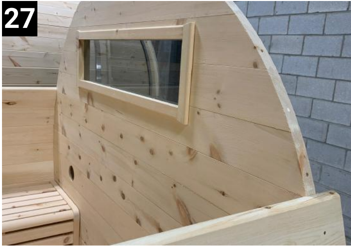
27 Add rest of back wall and fasten with 4" screws
