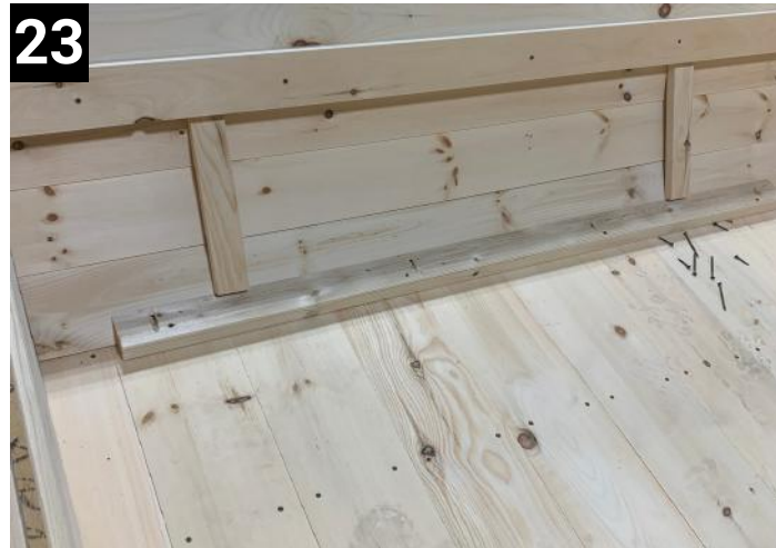
Using bench height measuring sticks fasten Ben h support cleat
