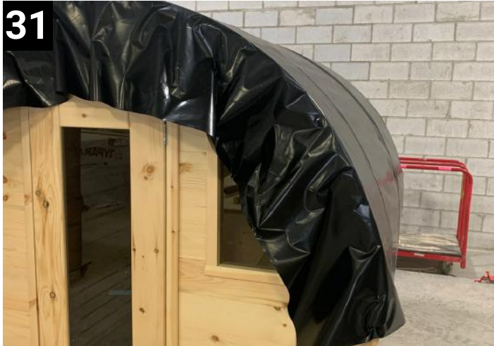
31 Put roof membrane over and make it even down both side. Staple over front staves
