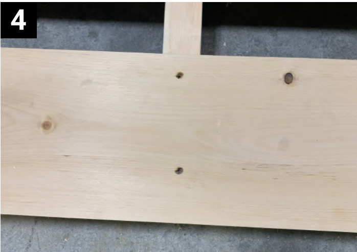
4 2 screws into each floor base. Leave Center long board with no screws. Walk isle area.
