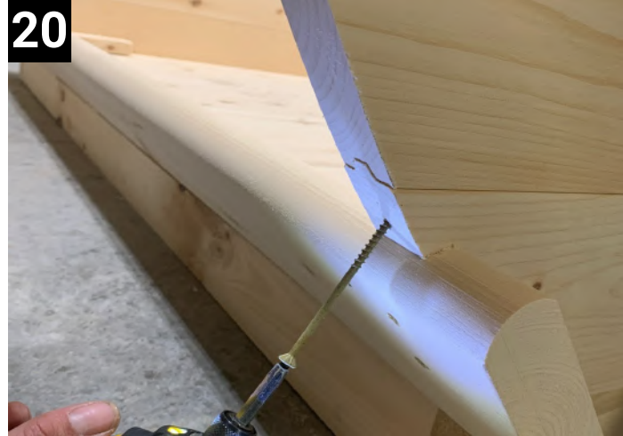
Screw wall together with a 4" screw
