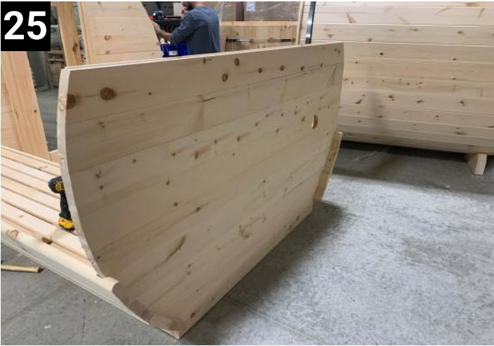
25 Add next back wall portion and fasten with 4" screws
